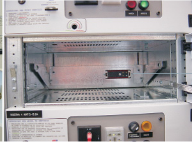
Combination of signal and power contacts in a slide-in system
