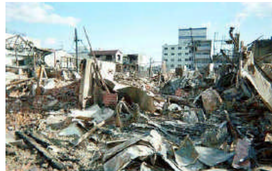
Figure 1: Disaster zone after an earthquake
