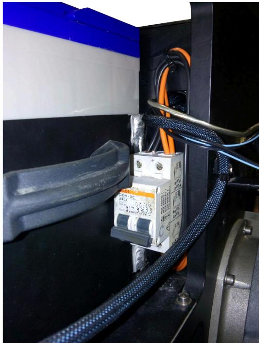
Figure H.4: Mounted circuit breaker.
